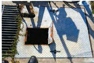
Inspection manhole
